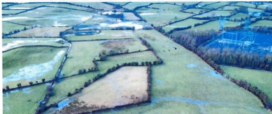
A view towards the northwest of site, where the drains are at high levels.
