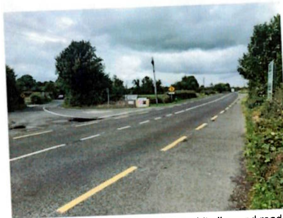
Photo 05: View to the north illustrates the continuous white line and road alignment.
