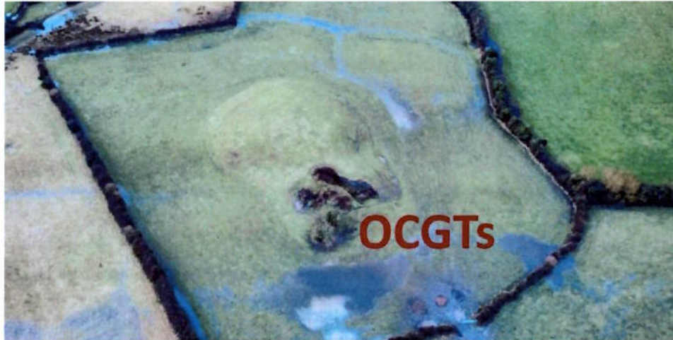
View of the site just south of the existing substation, where the 1,155 MW OCGTs are proposed to situate.
